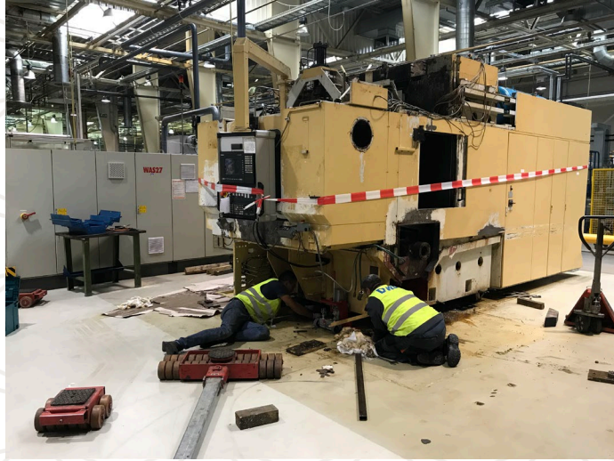
Dismantling – 8 MACHINES HOSBERG MACH 500 GERMANY
